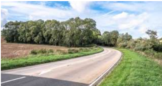
Approach from the south
